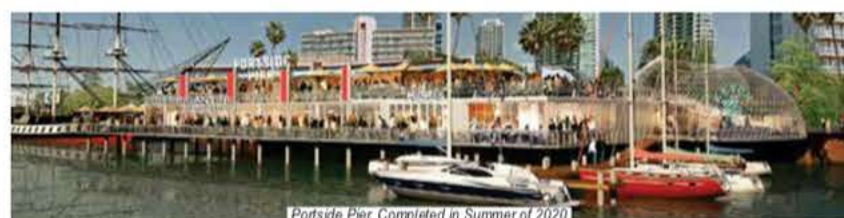
Portside Pier, Completed in Summer of 2020
