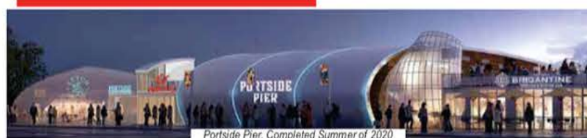
Portside Pier, Completed Summer of 2020
